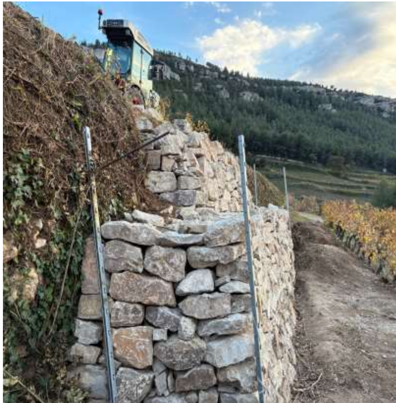
Figure 2. Rehabilitation of a dry-stone terrace breach at Domaine du Paternel (Cassis, France)
